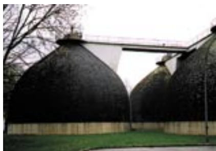
Figure 1: Standard sludge digestion of the Heidelberg sewage plant.
