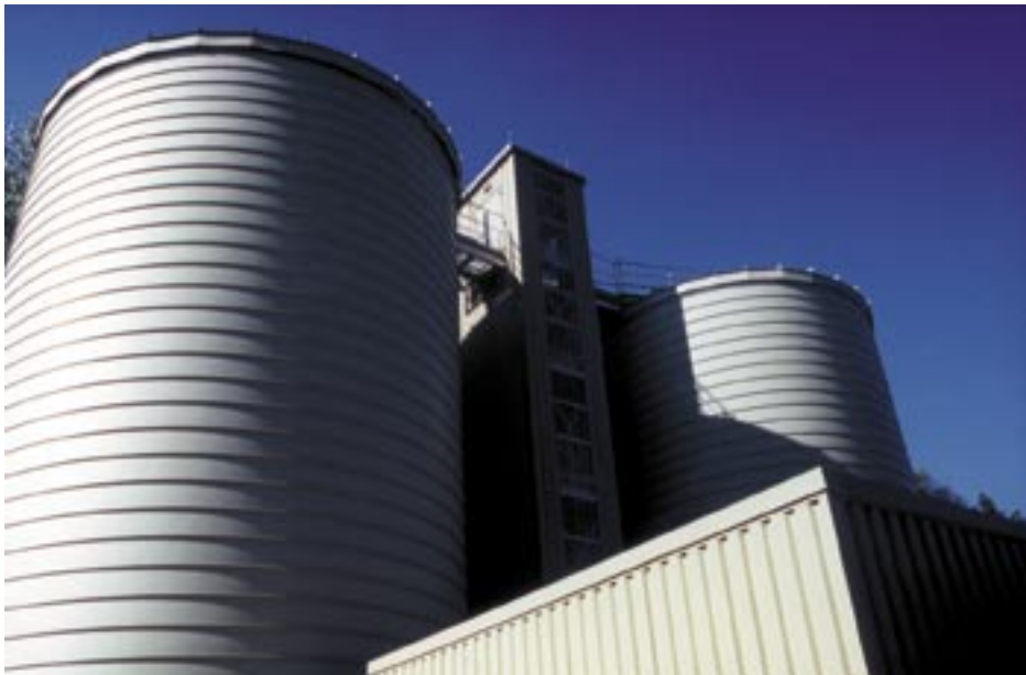
Figure 3: Two-step high-performance plant for the digestion of sewage sludge in Leonberg.
