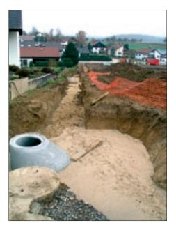
Figure 2: As part of the development work the wastewater infrastructure in the new settlement is being erected.
