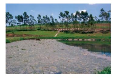
Figure 2: View of a wastewater lagoon established as decentralized treatment plant. Disadvantages of this processes are particularly for urban structures, the large amount of space, and the occasional odor pollution caused by overloading.
