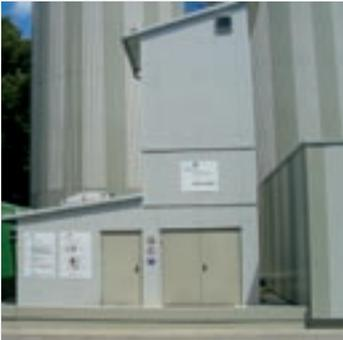
The Fraunhofer IGB has developed a sludge fermentation process, whereby integrated microfiltration enhances the decomposition of the sludge, and ammonium is recovered from the filtered sludge water. A pilot plant – consisting of a bioreactor, rotating disk filter and ammonia stripping plant – came online in 2004 as the second stage of a high-performance digestion of the Heidelberg Municipal Association for Sewage Treatment (*Abwasserzweckverband*).
