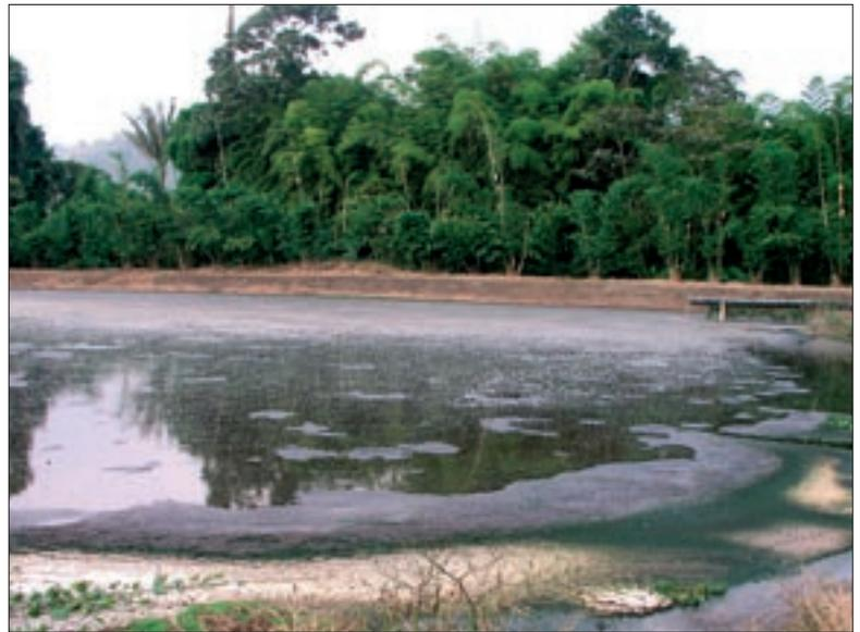
**Figure 4:** Simple biofilter unit for the treatment of wastewater from a sausage factory.
