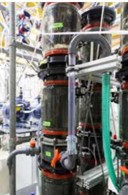
top: One-stage high-load digestion plant in Ilsfeld
